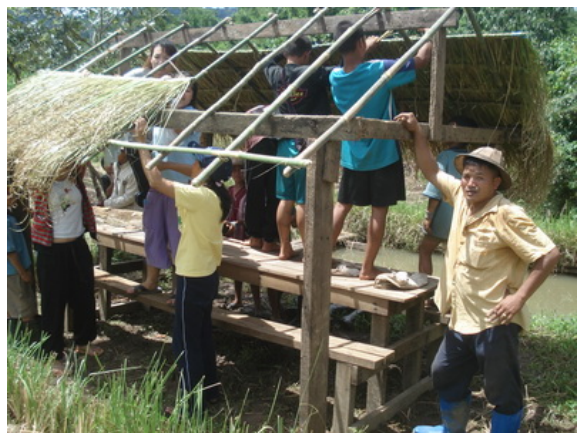
FIG.12 USE OF VETIVER THATCHING FOR ROOFING.
